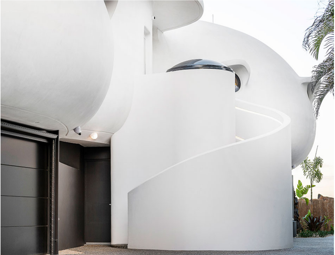
An organic design sees the home in conversation with the surrounding landscape, using a language of curves rather than angles. Design by Raunik Design Group, photo by Rezolution Photography, all rights reserved.
