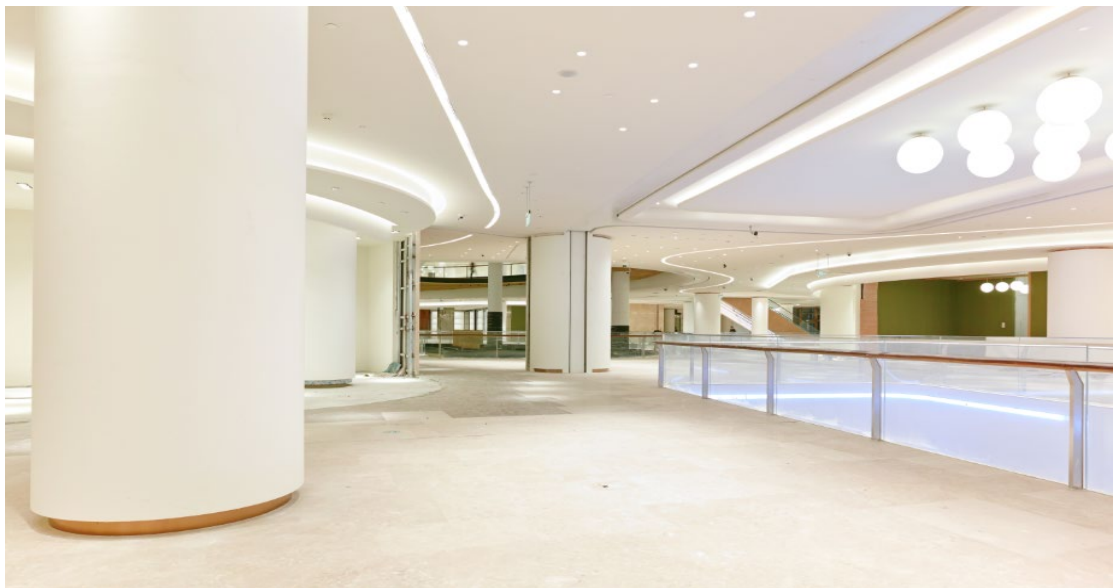
Mall interior cladding, column cladding, elevator hall, and retail shop countertops all made use of Corian® Solid Surface. Copyright material of DuPont™ Corian®
