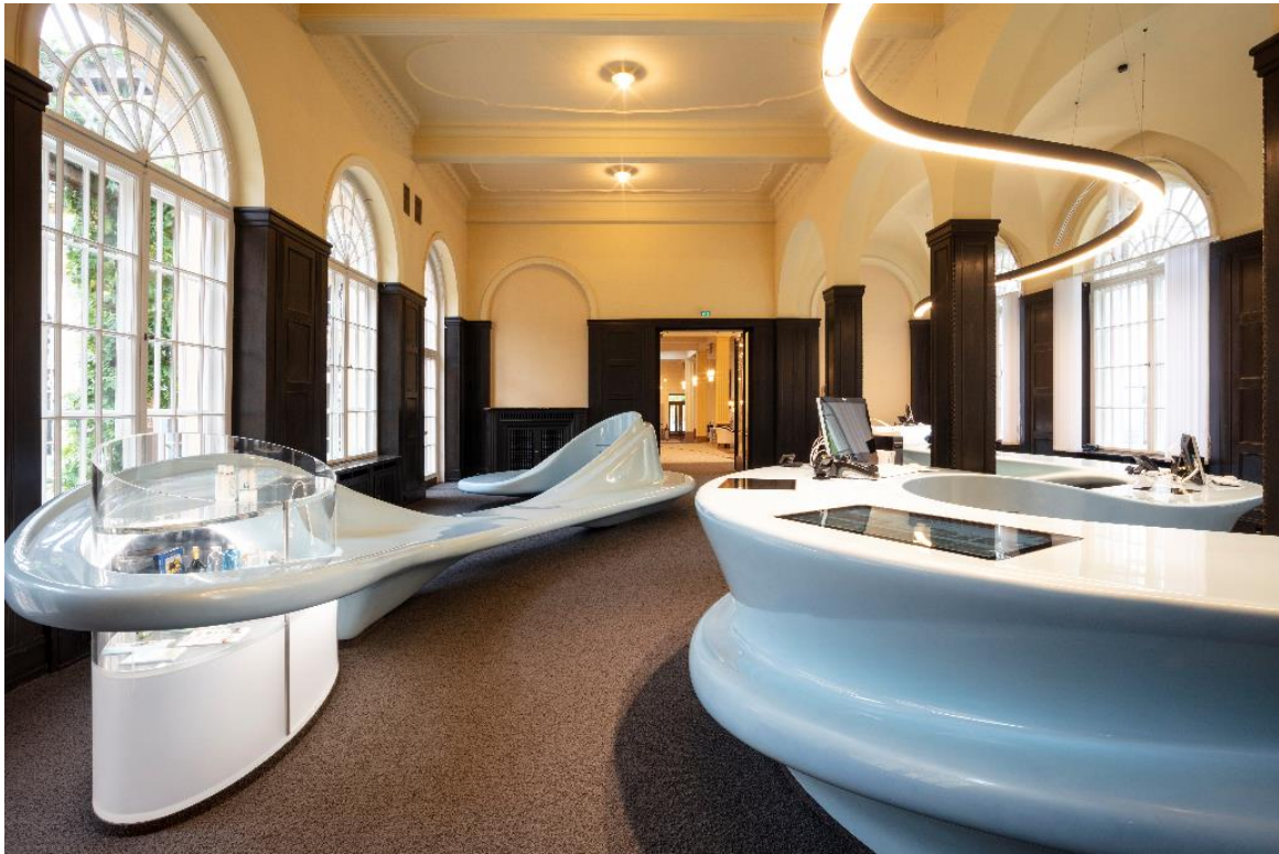
The counters of the Bad Kissingen Tourist Information centre were created on behalf of Bayerisches Staatsbad Bad Kissingen GmbH, and, thanks to the expertise of companies Grabner Design and Moser GmbH, are assembled from 4500 components made of Corian® Solid Surface. Concept / project / implementation: archicult - breunig architekten, Photo: Michael Stephan, all rights reserved.
