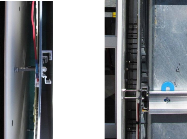
Figure 4: Side view images of the mounting system of a backlit panel before install and panels mounted on the garden wall.
