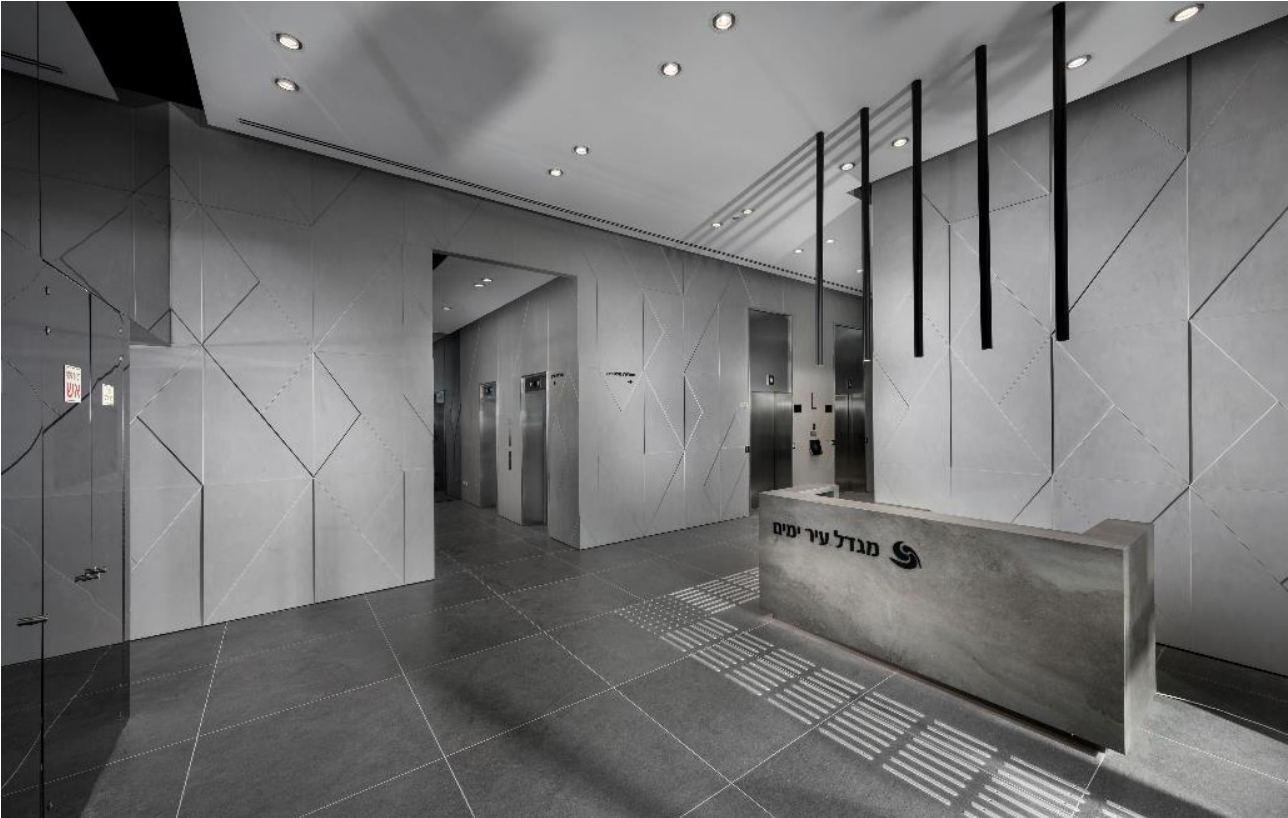
View from the park entrance - to the lobby features a reception area with wall cladding made with 3D geometric panels of Corian® Solid Surface in the recently introduced Neutral Concrete colour; project by MYS Architects; photo by Elad Gonen, all rights reserved.
