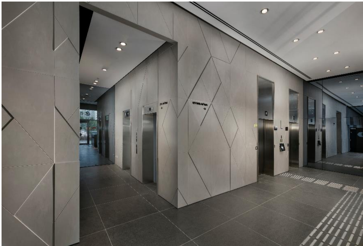
Ir Yamim high-rise office tower in Netanya, Israel: the lobby features a reception area with wall cladding made with 3D geometric panels of Corian® Solid Surface in the recently introduced Neutral Concrete colour; project by MYS Architects; photo by Elad Gonen, all rights reserved.
