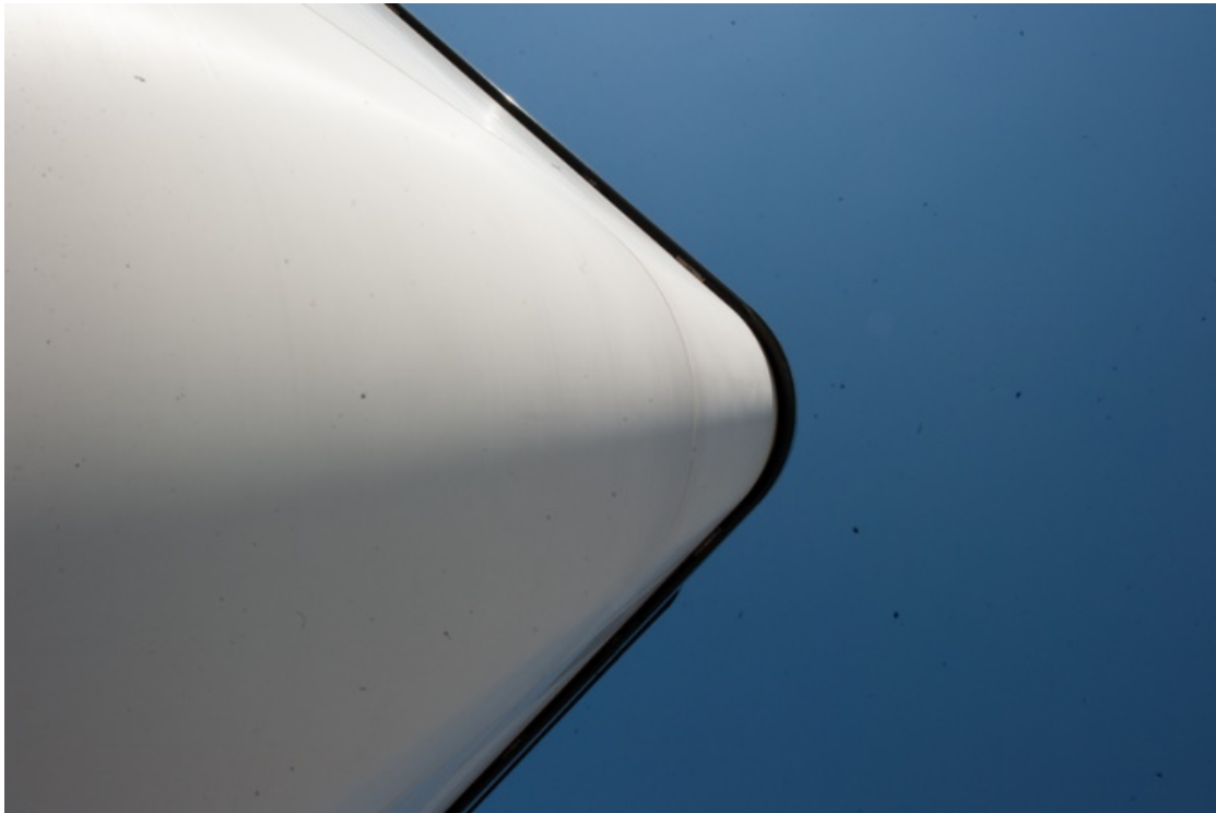
The "Glazialhaus" in Hamburg with a facade made of DuPont™ Corian® in colour Glacier White, Photo: www.behringstrasse126.de , all rights reserved.
