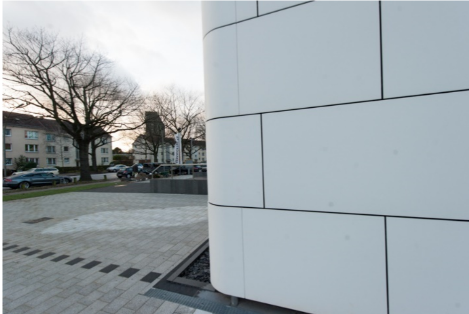
The fine, black seams of the facade made of DuPont™ Corian® in colour Glacier White yield an equally modern and timeless look for the “Glazialhaus” in Hamburg, Photo: www.behringstrasse126.de , all rights reserved.
