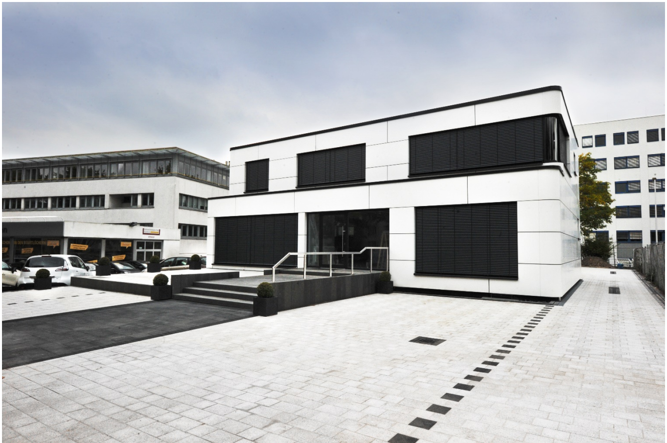
The “Glazialhaus” in Hamburg is clad with a facade made with DuPont™ Corian® in colour Glacier White, Photo: www.behringstrasse126.de , all rights reserved.
