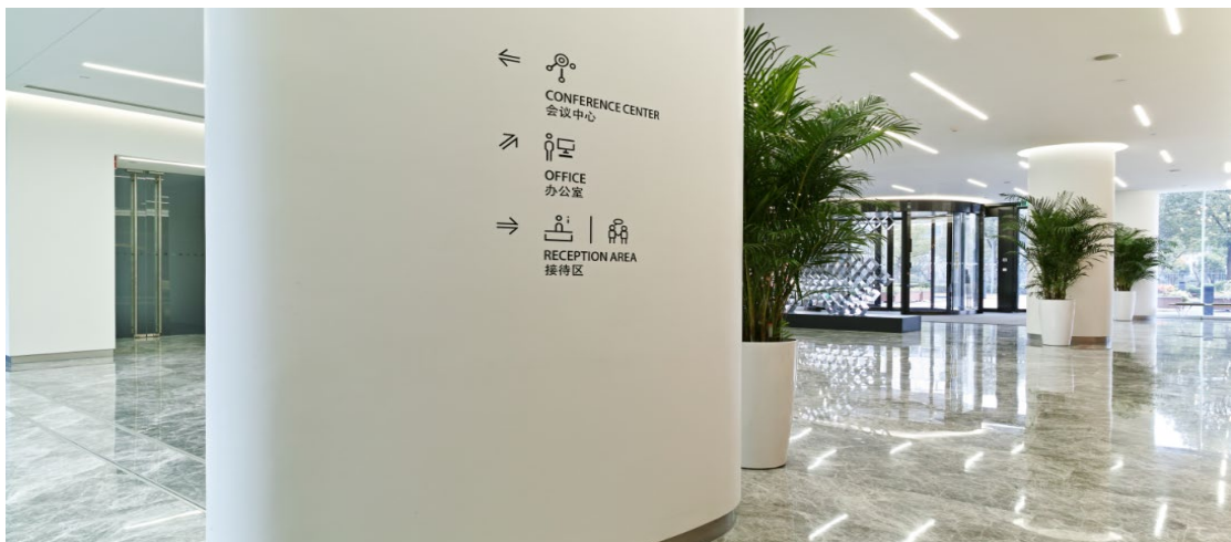
Corian® Solid Surface glacier white used in the seamlessly covers the lobby pillars. Photography by Fang Yuan.
