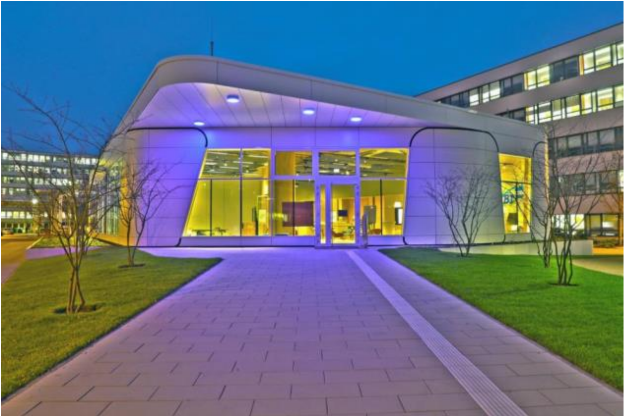
Ingelheim am Rhein, Germany, headquarters of Boehringer Ingelheim: the BI CUBE featuring a façade made with Corian® Exteriors panels, a solution based on Corian® Solid Surface; project by Hirschmuellerschmidt Architektur; photo courtesy of Boehringer Ingelheim, all rights reserved.
