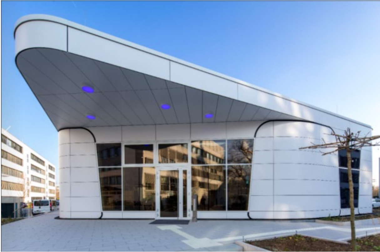
Ingelheim am Rhein, Germany, headquarters of Boehringer Ingelheim: the BI CUBE featuring a façade made with Corian® Exteriors panels, a solution based on Corian® Solid Surface; project by Hirschmuellerschmidt Architektur; photo courtesy of Boehringer Ingelheim, all rights reserved.
