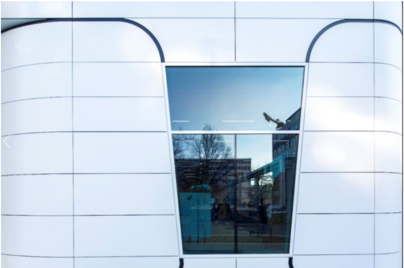
Ingelheim am Rhein, Germany, headquarters of Boehringer Ingelheim: the BI CUBE featuring a façade made with Corian® Exteriors panels, a solution based on Corian® Solid Surface; project by Hirschmuellerschmidt Architektur; photo courtesy of Boehringer Ingelheim, all rights reserved.
