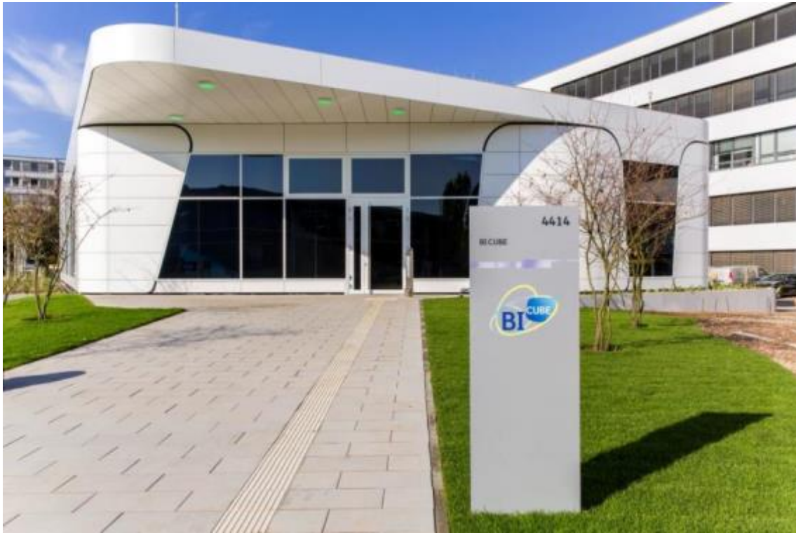
Ingelheim am Rhein, Germany, headquarters of Boehringer Ingelheim: the BI CUBE featuring a façade made with Corian® Exteriors panels, a solution based on Corian® Solid Surface; project by Hirschmuellerschmidt Architektur; photo courtesy of Boehringer Ingelheim, all rights reserved.
