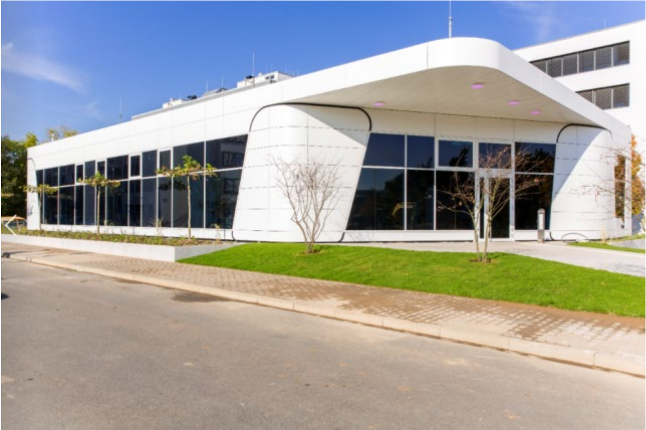
Ingelheim am Rhein, Germany, headquarters of Boehringer Ingelheim: the BI CUBE featuring a façade made with Corian® Exteriors panels, a solution based on Corian® Solid Surface; project by Hirschmuellerschmidt Architektur; photo courtesy of Boehringer Ingelheim, all rights reserved.
