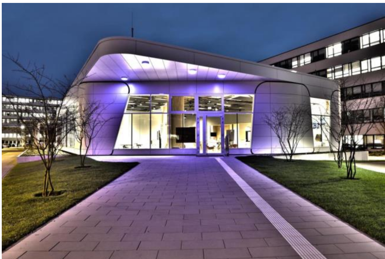
Ingelheim am Rhein, Germany, headquarters of Boehringer Ingelheim: the BI CUBE featuring a façade made with Corian® Exteriors panels, a solution based on Corian® Solid Surface; project by Hirschmuellerschmidt Architektur; photo courtesy of Boehringer Ingelheim, all rights reserved.
