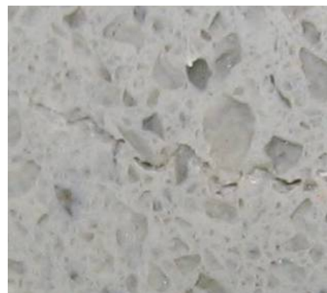
Surface Crack
